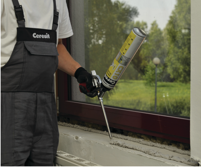
Foam application for window sill installation
