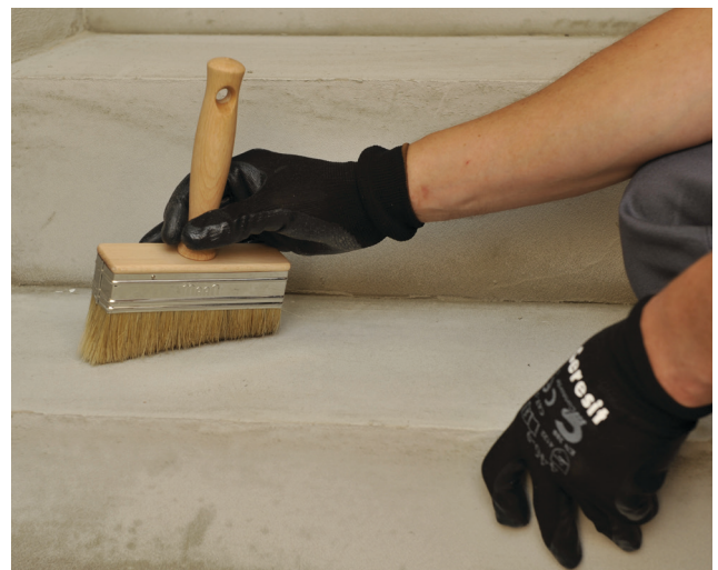
Cleaning the substrate
