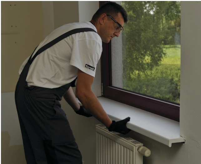
Window sill installation and stabilization
