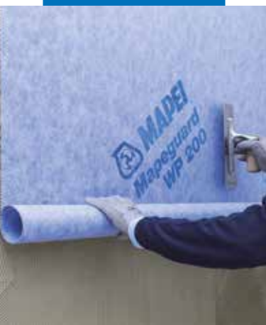
Instalace fólie Mapeguard WP 200
