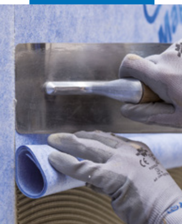
Application of the second sheet
