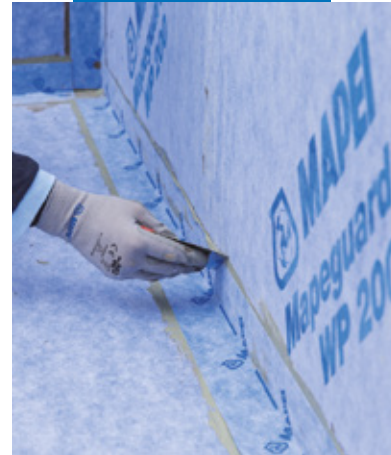
Application of Mapeguard ST
