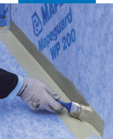
Application of the Mapeguard WP Adhesive in order to seal the joints in the corner before the application of Mapeguard ST
