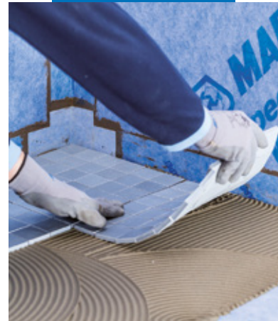
Laying of the tiles
