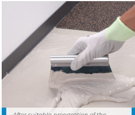
After suitable preparation of the substrate, spread on the adhesive to bond the soundproofing sheets
