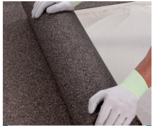
Unroll the sheets of Mapesonic CR on the surfaces to be soundproofed
