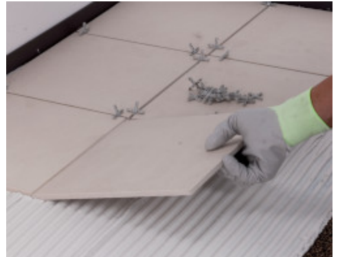
Spread the adhesive on the Mapesonic CR and bond the new floor finish
