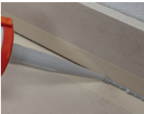
Seal the gap between the skirting board and the floor with a suitable flexible sealant from the Mapei range
