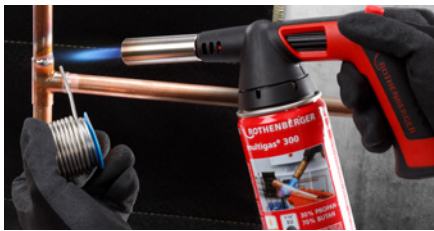
Soft soldering in drinking water and heating installation
